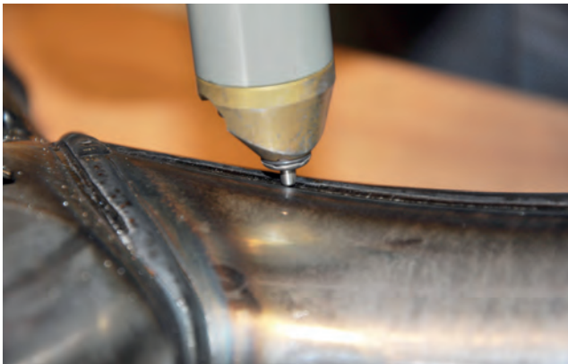
Figure 15: Ultrasonic needle peening of the weld toe
